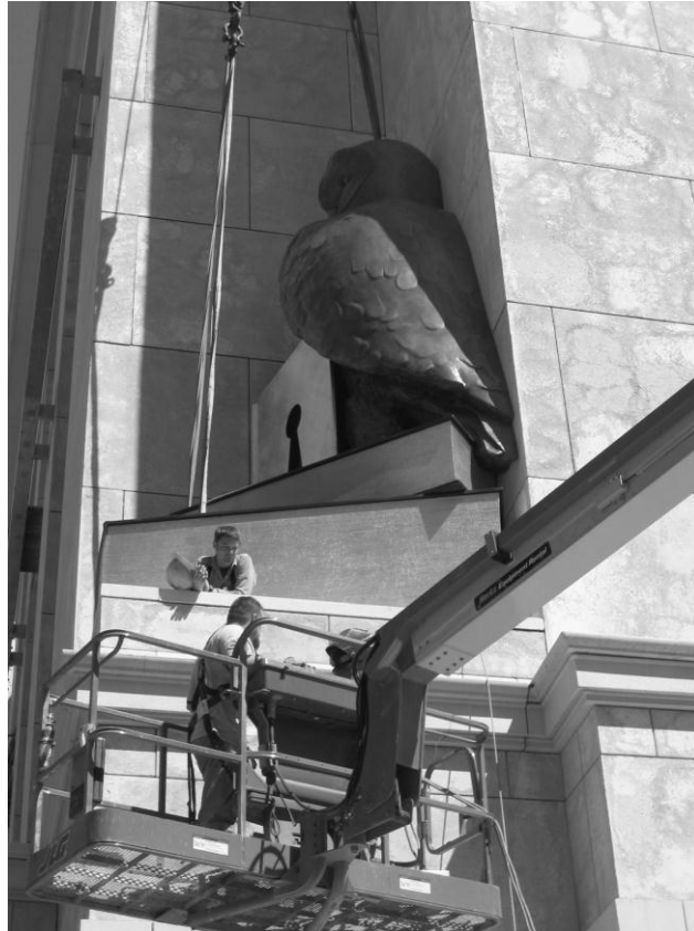
Installation of Wisdom exterior of Main Library, Jacksonville, Fla., 2005
